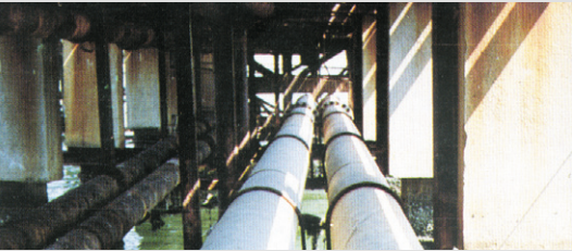
Deck steam drain pipe, 13 years in use AFTER 13 YEAR OF SEA WATER DRAN PIPE (130M FROM SEA WATER INLET)
